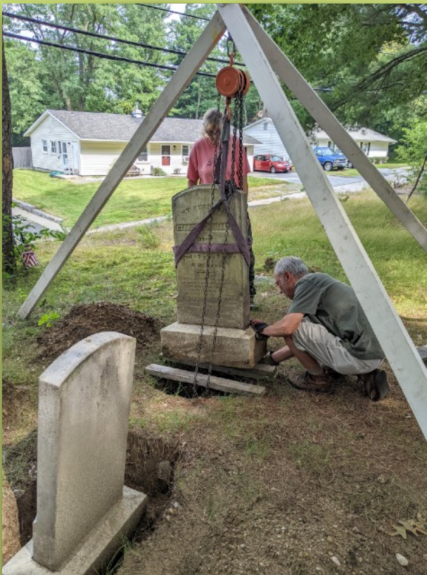
Ed Walker demonstrates how to position the headstone.
