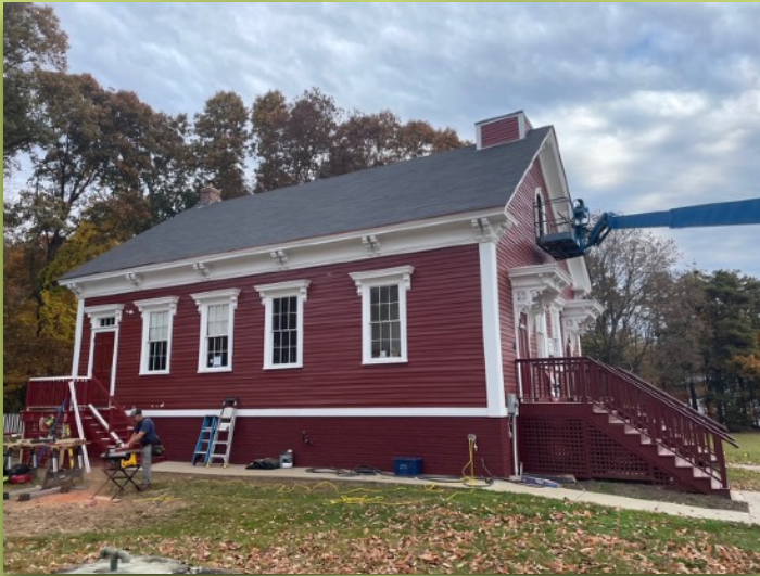
A new cupola base has been installed
