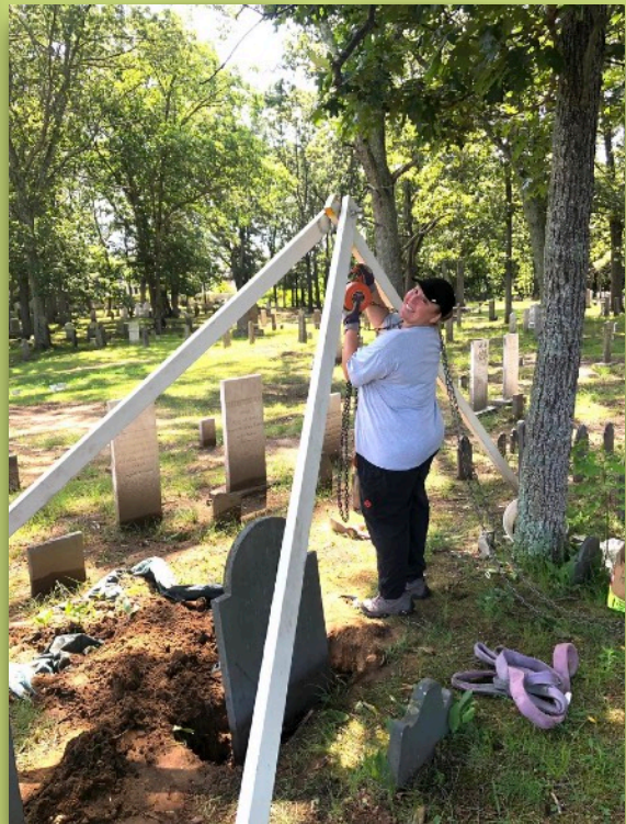
Stephanie is setting up a hoist for lifting heavy headstones.
