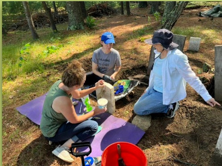
Julie, Hannah and Audrey work to repair a foot stone.
