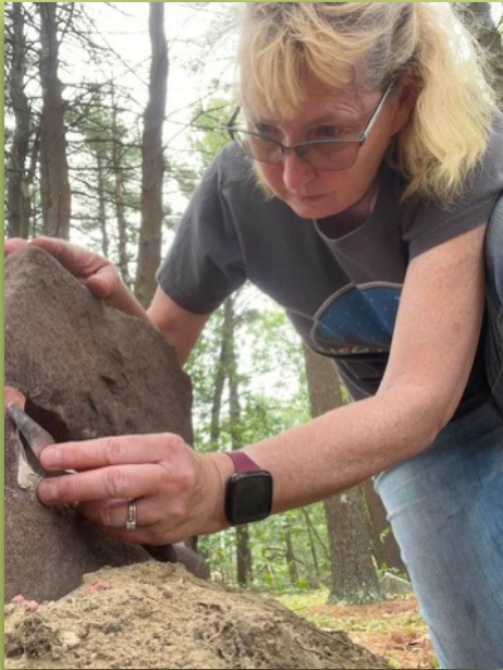
Kim is applying infill to a crack in a gravestone.
