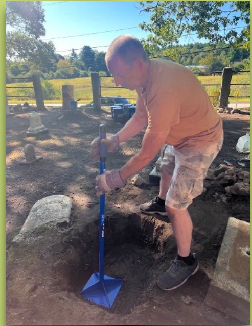
Gene Baillargeon preparing a firm and level foundation for a base.
