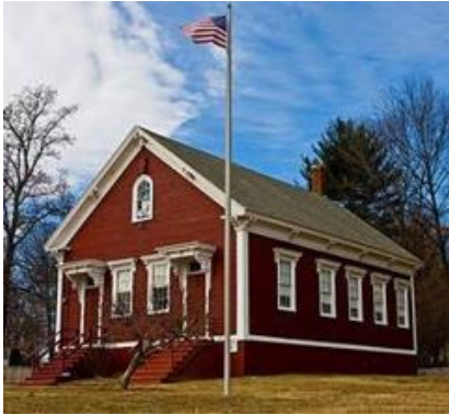
Forestdale One Room Schoolhouse - 1877 190 School St., Forestdale, RI (leased by NSHA from the Town)
